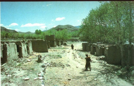
Within the broken buildings along the village's main street, returning guerrillas hide out
